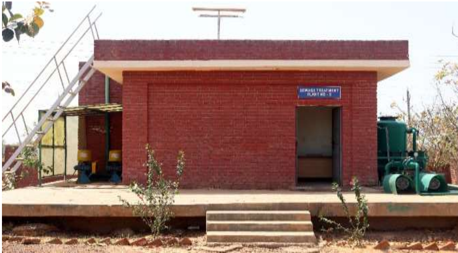
Sewage Treatment Plants (STP) at the campus
