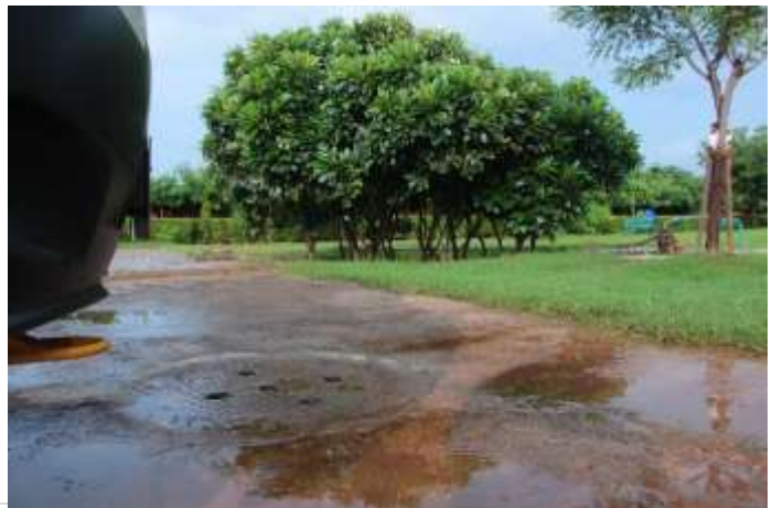
Rain Water Harvesting Pit (RWH), at the campus
