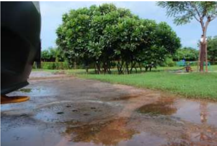
Rainwater Harvesting pits at different locations in the campus
